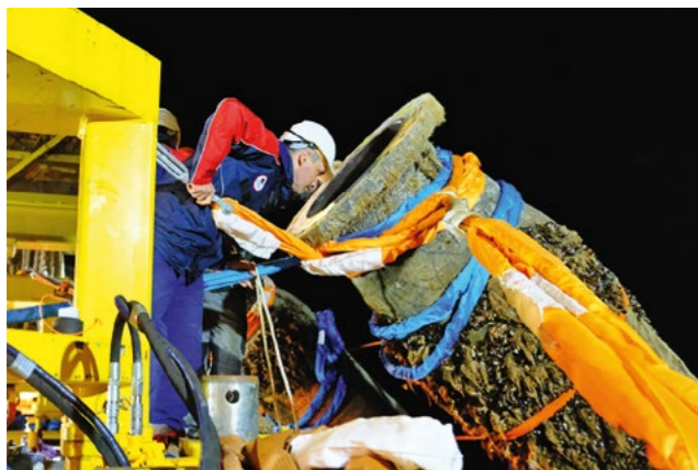
Replacement of the MLBs' buoyancy tanks at the Marine Terminal. 2022
