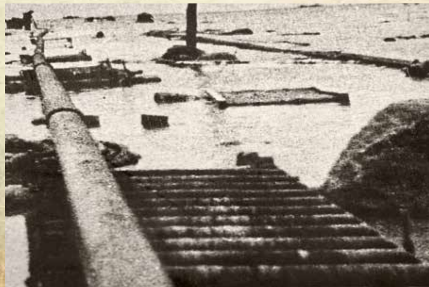
LAYING OF THE KAREJA-BORISOVA GRIVA PIPELINE ALONG THE BOTTOM OF LAKE LADOGA IN THE SPRING OF 1942
