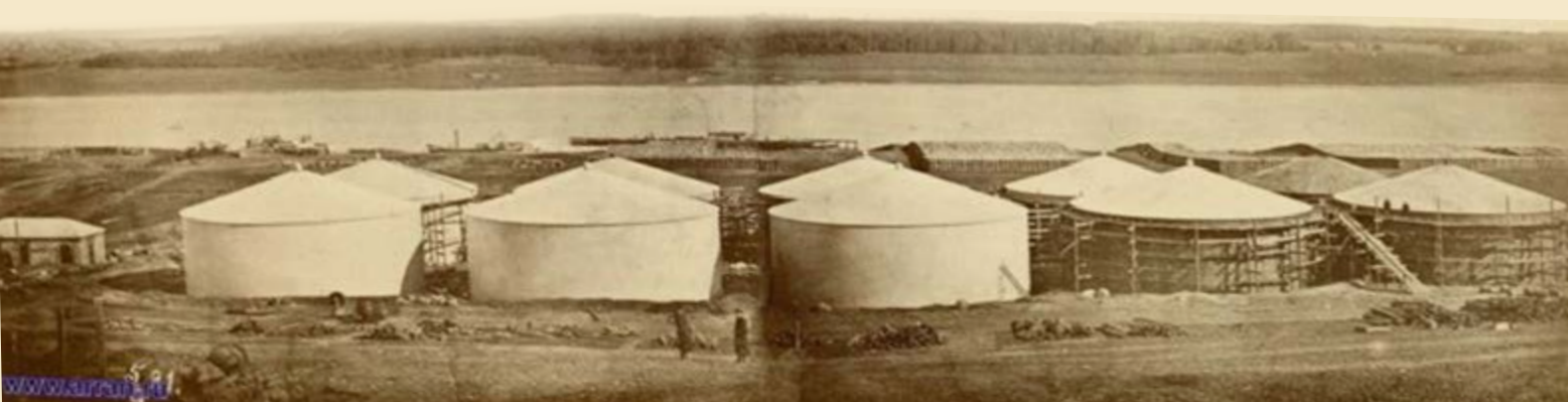
Tank Farm Construction Designed by V. G. Shukhov, Konstantinovka, 1881
