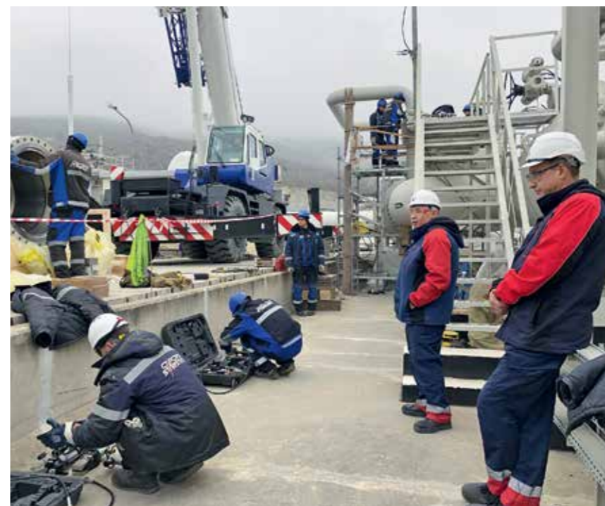
REPLACEMENT OF THE BALL VALVE, 2020
