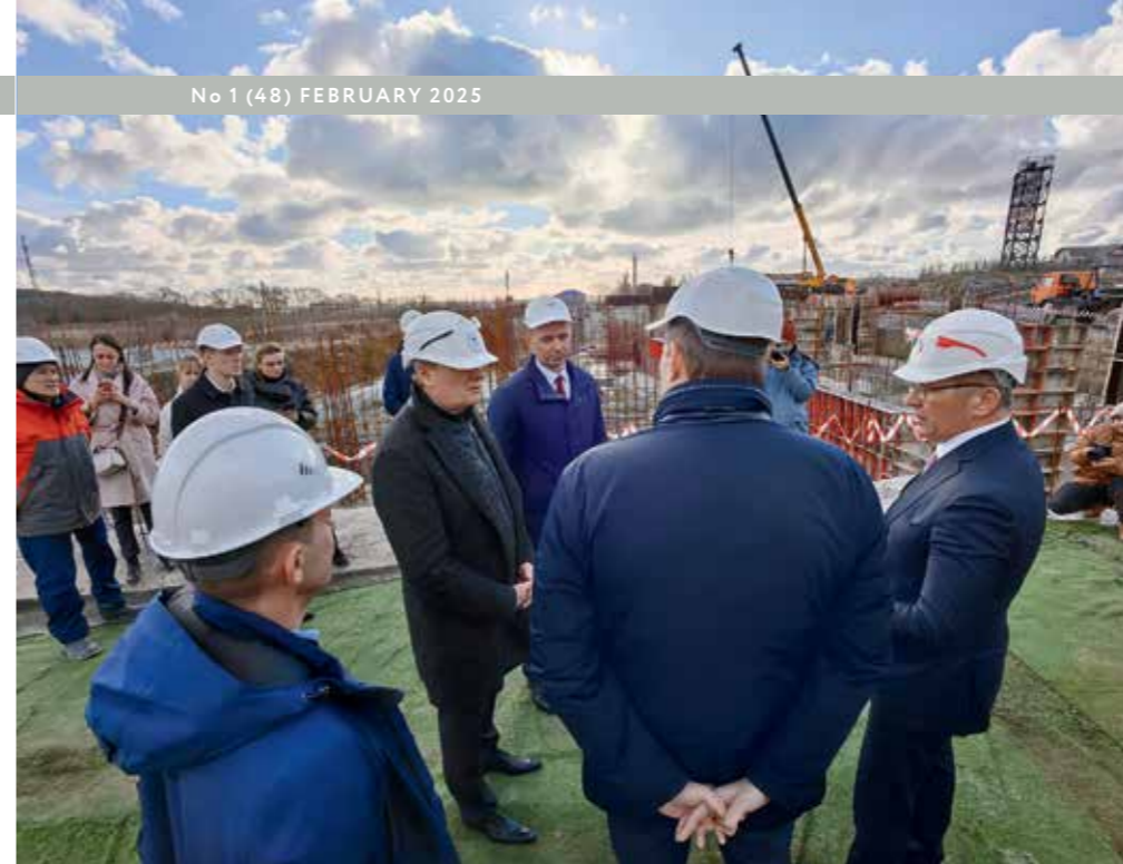
CONSTRUCTION OF THE CACCY IN YUZHNYAYA OZEREYEVKA
