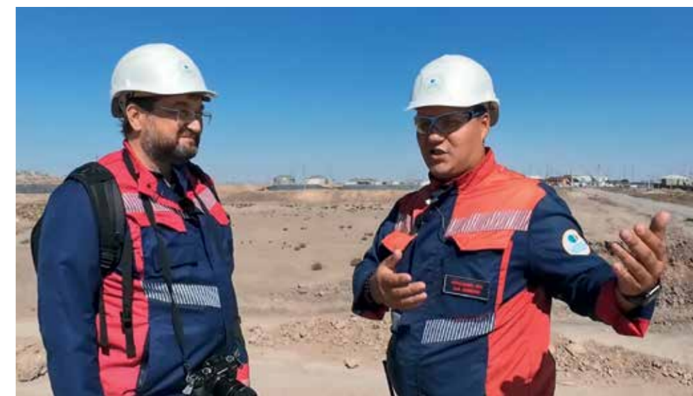
P.A. KRETOV AND D.M. AKHMETOV AT THE CONSTRUCTION SITE OF THE PROTECTIVE DAM
